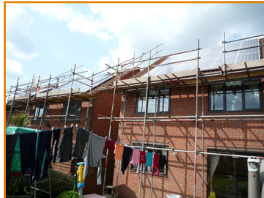
Three installations in progress
