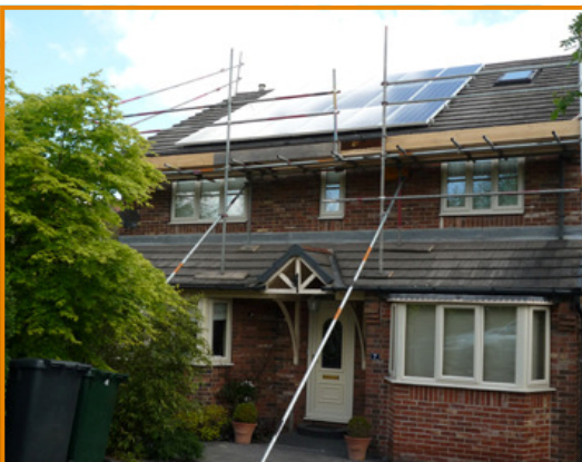
A typical installation in progress
