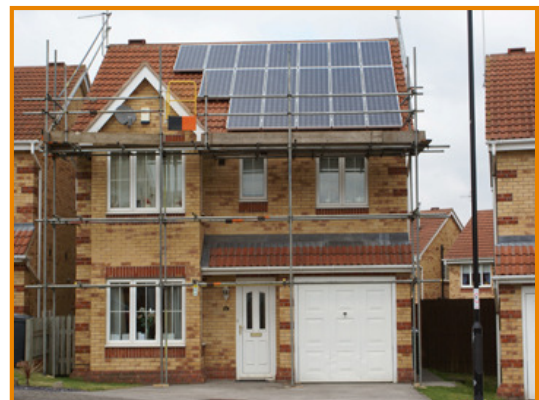
A typical installation in progress
