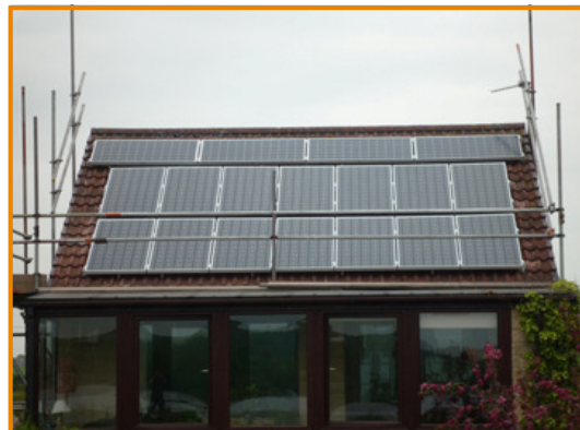
A completed installation
