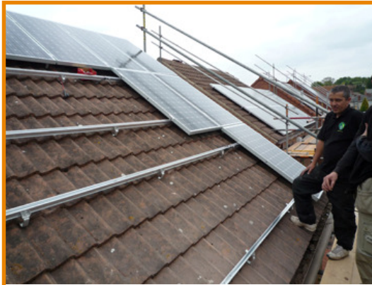
Solar panels being installed
